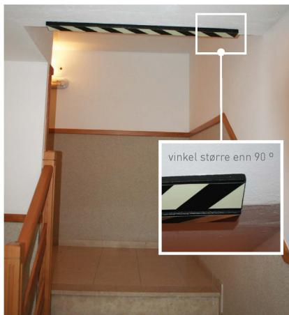
Støtdemper for flate overflater N 81 21
